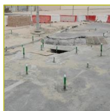
Injections in urban areas to reduce subsidence
