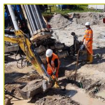
Large excavations & earthworks
