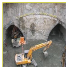
Traditional tunnel excavation
